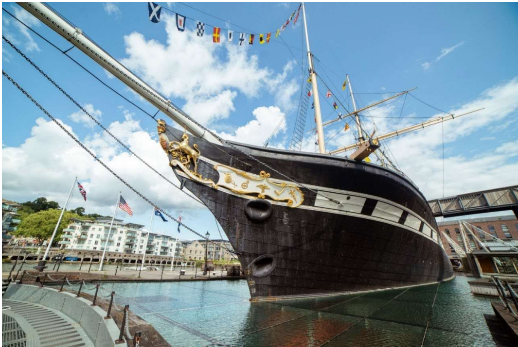
Figure 3: A seal at waterline level with a 50mm layer of water on the glass plate provides insulation while creating the appearance that the ship is ready to set sail.
