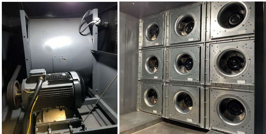
Figure 6: Belt-driven scroll fan (left, 2005-2021) replaced by a grid of nine direct-drive fans (right, 2022-present).
