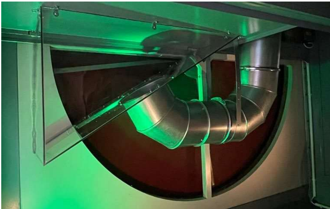
Figure 7: Energy Recovery Purge system fitted to the desiccant rotor on the dry dock dehumidifier.
