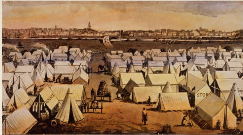
‘Canvas Town, between Princess Bridge & South Melbourne in 1850s’ (De Gruchy & Leigh, between 1850 and 1860). Tents put up in Melbourne to house new arrivals from Britain c. 1852 | State Library Victoria
