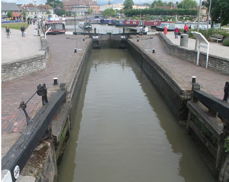
A typical river or canal lock at Stratford upon Avon. In this case the gates are operated by hand. The ones nearest the observer are open, the others are closed.
