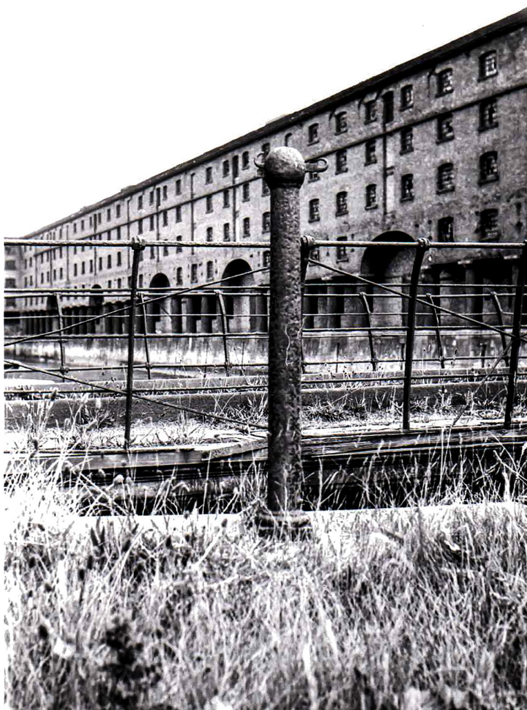
Albert Dock in Liverpool was derelict from 1972 to 1983. The site had many interesting features including the cast iron double leaf swing bridge in the middle ground, which needed subtlety in its restoration.
