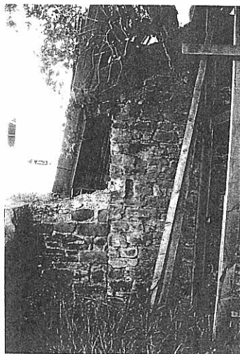
[45] Walling, possibly 1840s, projecting off the S boundary masonry wall & containing a blocked stone arch.
