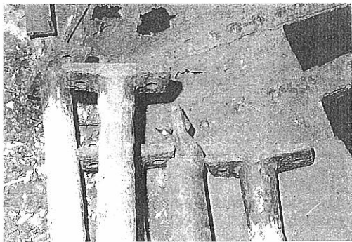
[81] Loose stanchions in the ship in 1998 clearly show the design of the stanchion base (although there are variations to the stanchions in situ) and the curved lapped design of the top which curves over the bulb to support the Butterley beams.
