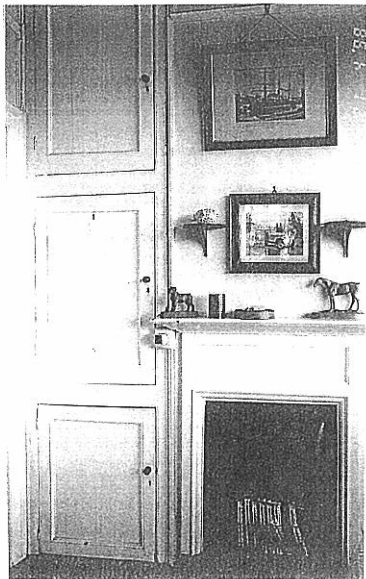
[30] Stylistic evidence - the small panes of the oriel window and the joinery in the office suggests a date of c. 1840
