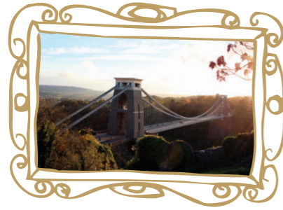
Clifton Suspension Bridge
